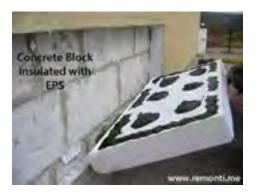
**EPS foundation insulation:** Installers glue masonry-faced EPS-foam sheets to the block wall.
