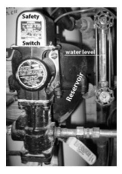
Sight glass & low-water control: The sight glass shows the boiler water level. The low water control adds water to the boiler and extinguishes the burner if the water level is too low.
