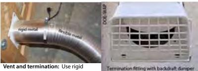
Vent and termination: Use rigid metal vent pipe if at all possible. Or use flexible metal vent and not foil vent when flexibility is required.
