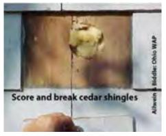
Score and break a shingle: If the shingles are flexible, you may be able to remove nails. However, usually you must score and break the shingle, and then later facenail it back in place.
