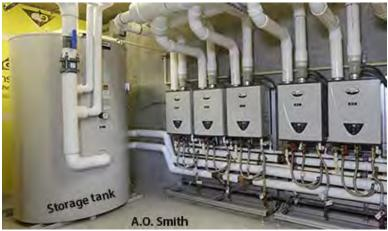
**Popular multifamily water-heating solution:** On-demand water heaters heat water for a storage tank and for demand in a medium-sized multifamily building.
